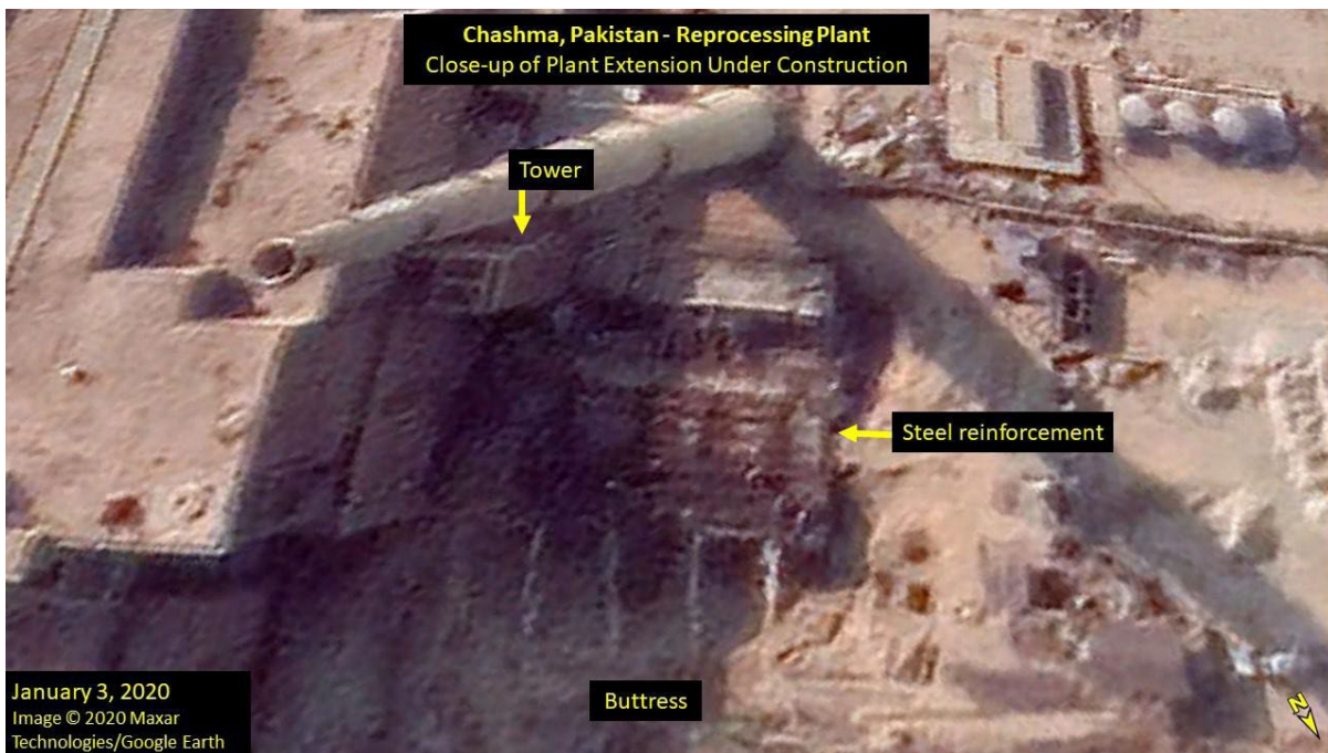
Image. More than a year later, in January 2020, construction of the extension has progressed in height with steel reinforcement.
