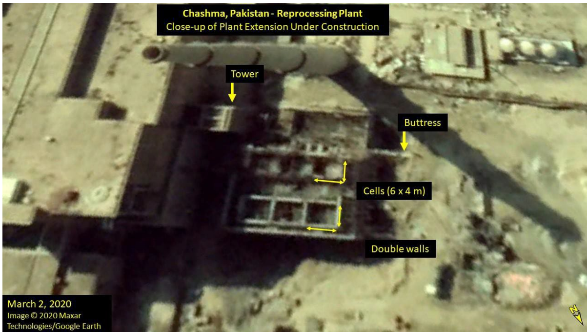
Image. In this March 2020 Google Earth image the layout of one of the upper stories is visible: six cells with double concrete walls, and a hallway.
