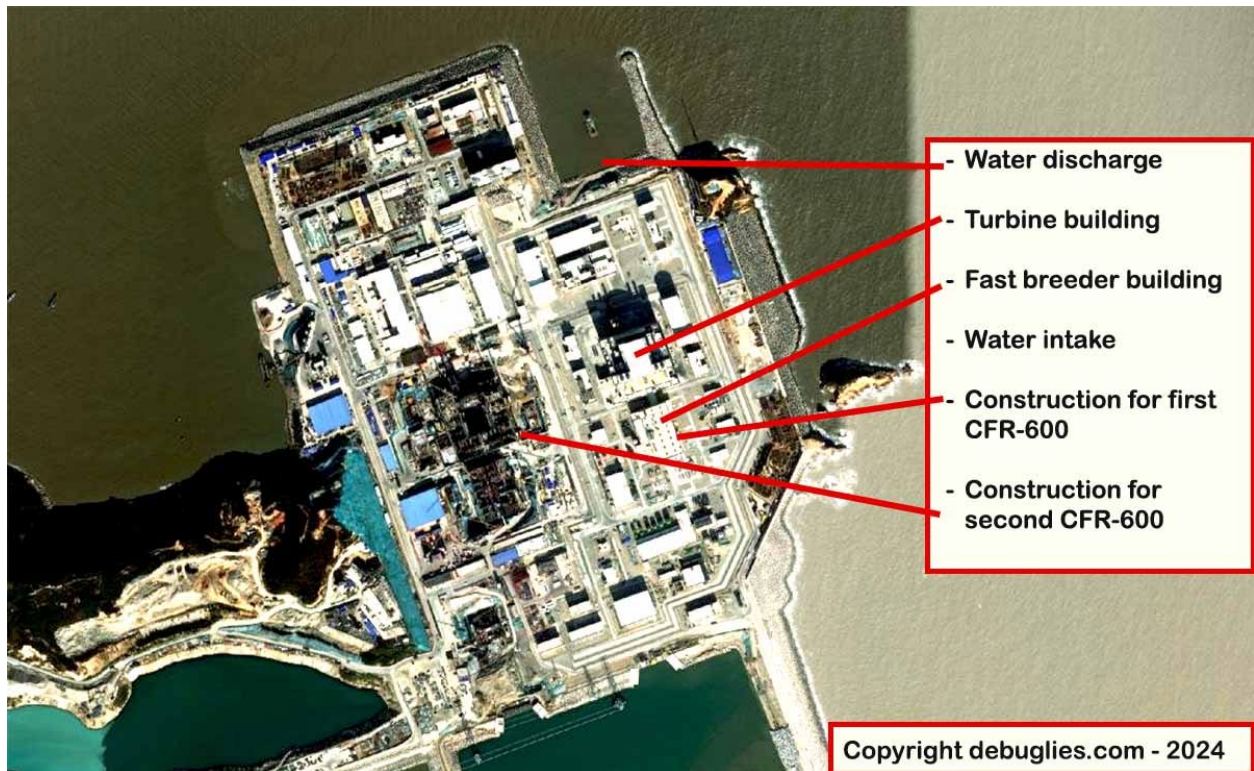
Image : Satellite imagery showing construction progress of the CFR-600 fast breeder reactors at Xiapu in Fujian province, China
