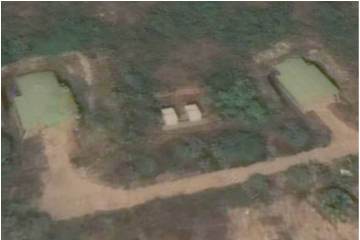
Image: The INS Varsha naval base under construction near Rambilli, India – copyright debuglies.com
