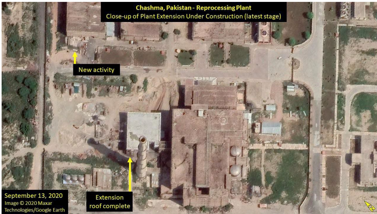
Image. The extension is externally complete in September 2020.
