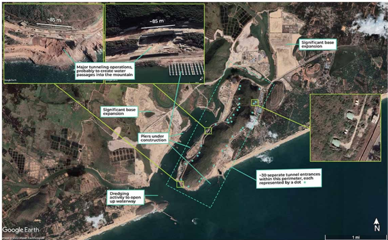
INS Varsha Naval Base Under Construction, Rambilli February 2022 / 17.4391, 82.8886
